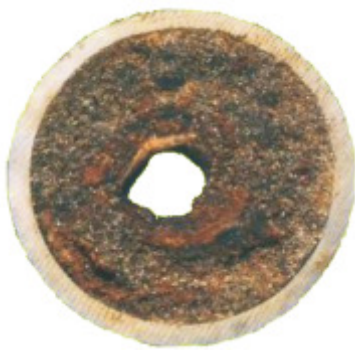
Lateral cut of a pipeline with extreme paraffin deposition
